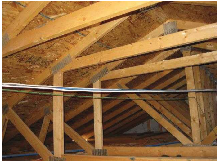
Garage attic view
