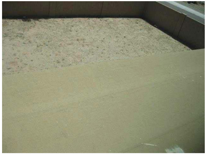
Patio roof view
