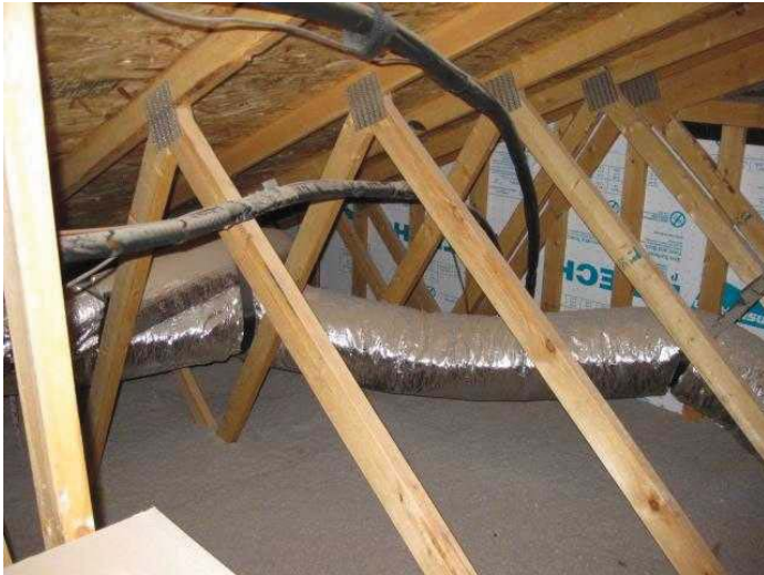
Upstairs attic view
